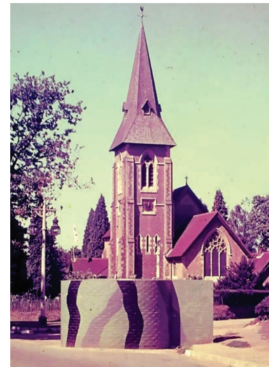
The Great Wall of Whitmore. We don't know exactly what this structure was for. It's made of brick, camouflaged, has ventilation pipes coming out of the roof and blocks the exit from Whitmore Vale Road. It's presumed to be part of a system intended to defend Crossways, although a single tank shell would have blown it to smithereens. The photo was taken by Stanley Beard.
